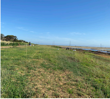
Revegetated horizontal levee
