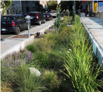
Green stormwater infrastructure
