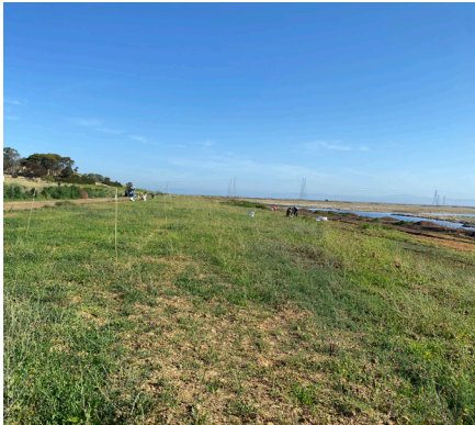
Revegetated horizontal levee
