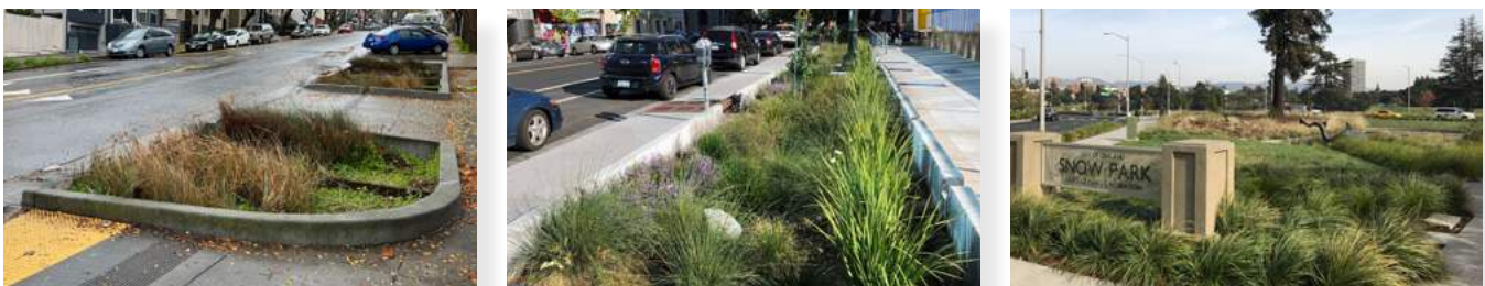
Green stormwater infrastructure in Oakland and San Francisco
